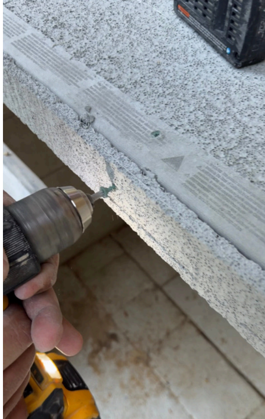
Fasten cement board without overdriving screws or breaking the edges.
